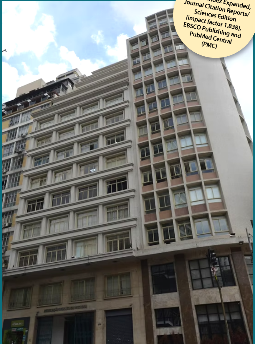
Associação Paulista de Medicina building, São Paulo city, State of São Paulo Photo: APM collection
